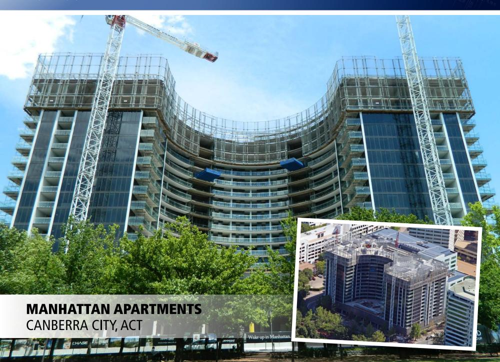
AFS LOGICWALL was specified on this project for vertical structural wall elements and secured a package for walls from Basement 2 to Level 16. AFS commenced delivery to the project on 29 March 2012 and continued delivering on a weekly cycle until the structure was complete on 29 November 2012.
