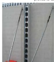
Ensure there is enough clearance to achieve the required concrete cover around the reinforcement bars that are to be installed through the created hole
