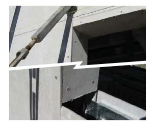
Large span lintels will need temporary propping during and after pour until adequate cure time has been reached. Refer to project structural engineer for advice.
