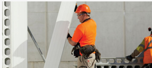
Step 1 Lightweight panels make for easier materials handling.
