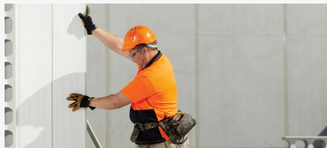
Step 3 And simply slide down to seat into the floor tracking and form a wall.
