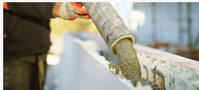
Step 6 Core filling.
